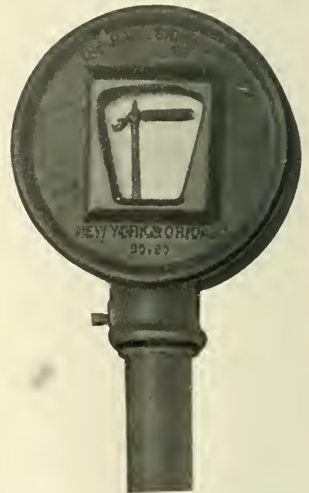
HALL AUTOMATIC SWITCH INDICATOR —LATEST TYPE.
